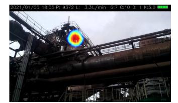
Compressed gas leak from the pipe in high place out of reach is found.
